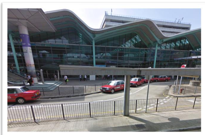
Outside Hung Hom MTR Station, Exit C
